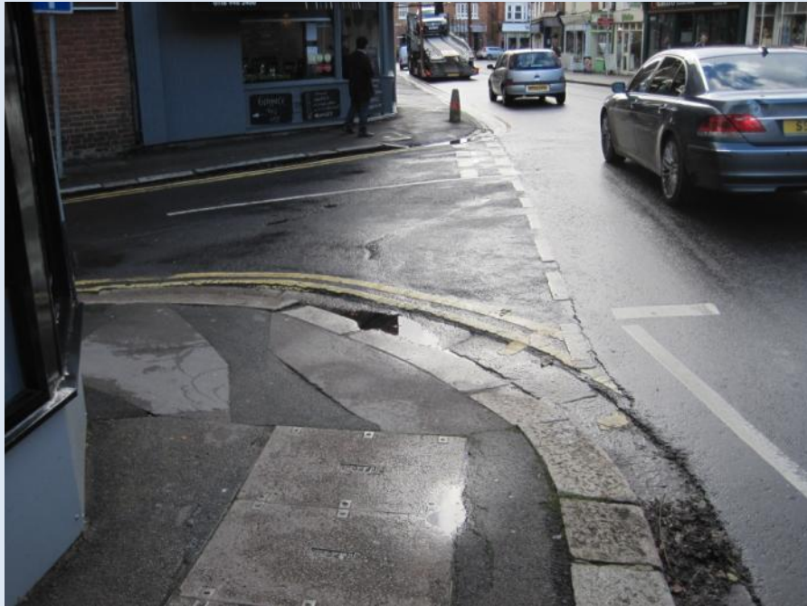
North Street Caversham
